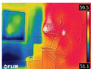
Uninsulated Outside Wall
