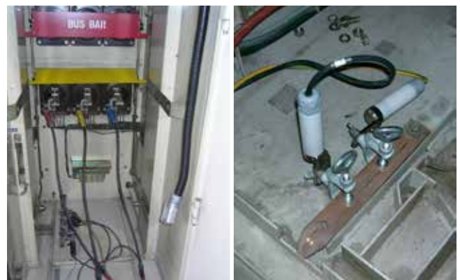
➤ 3 phased connection, common grounding point of safety earth and operation earth clamps
