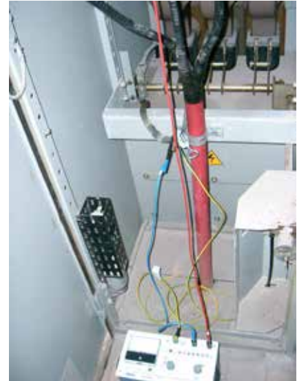
➤ galvanic connection of audio frequency generator TG
