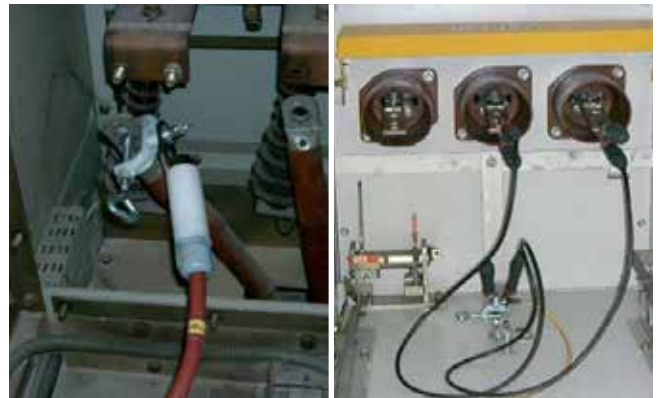
➤ single phased connection, not involved phases grounded
